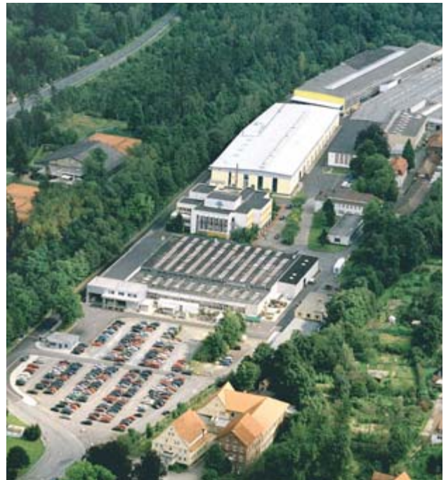
Piller Headquarters & Manufacturing Facility - Osterode
